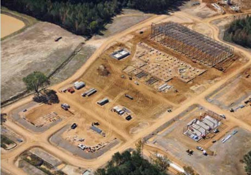
(Left) Mississippi Silicon is constructing a \$200 million silicon metal production facility on the Tenn-Tom Waterway in Tishomingo County. The main building is 150 feet high and has a 38-foot reinforced concrete foundation.
